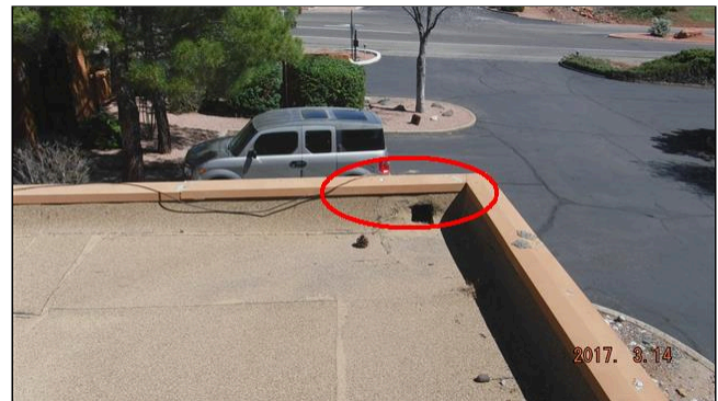
1.0 ROOF COVERING 1 (Picture 2) Roof Drain
