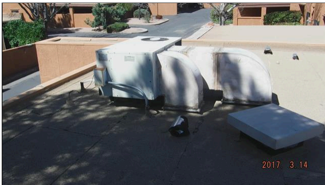
11.1 OUTDOOR UNIT WITH SAFETY SHUT OFFS (Picture 1)
