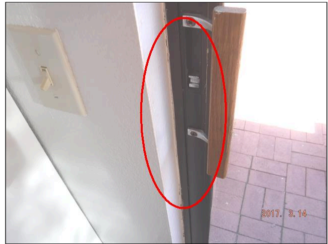
8.7 SLIDER/PATIO DOORS (Picture 1)
