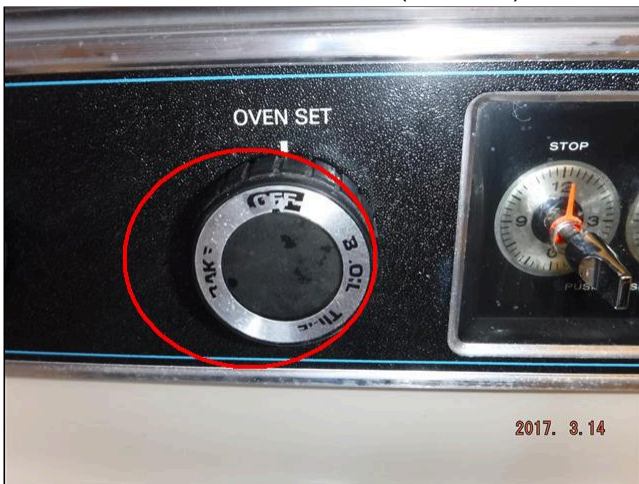
7.4 RANGE (Picture 2) Worn controls
