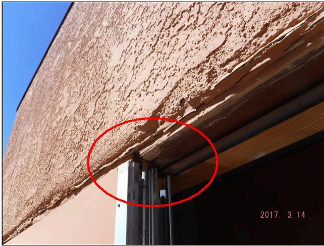
2.2 ENTRY DOORS (Picture 1)
