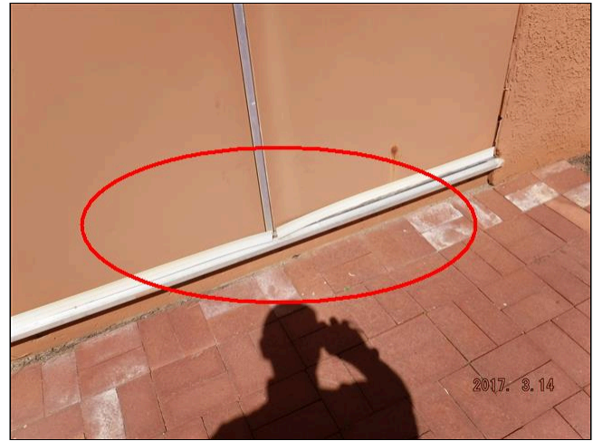
2.2 ENTRY DOORS (Picture 2)
