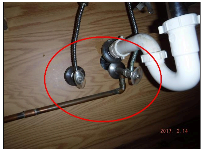
6.0 SINK(S)----- BATHROOM ONE (Picture 2)
