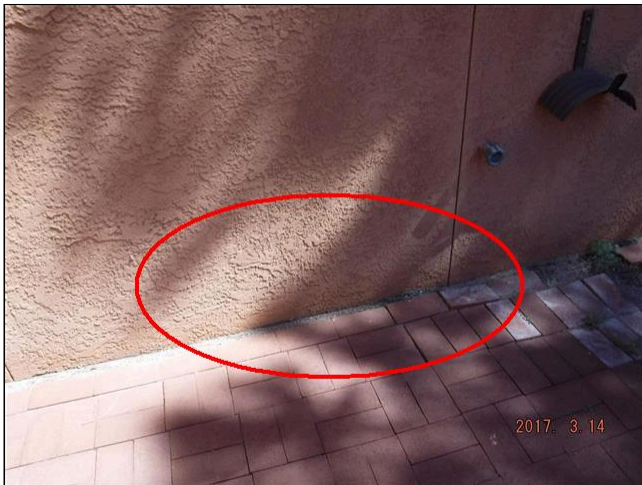
2.6 FOUNDATION COATING (Picture 1)
