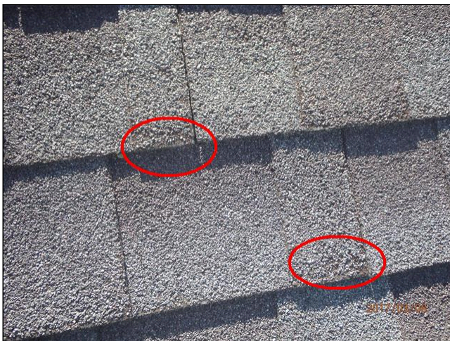
1.0 ROOF COVERING (.1) Item 1(Picture)
