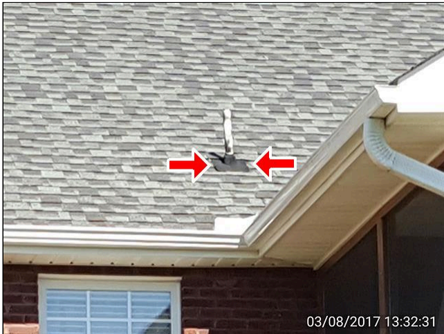
1.2 PLUMBING/ELECTRICAL STACKS (.1) Item 3(Picture)
