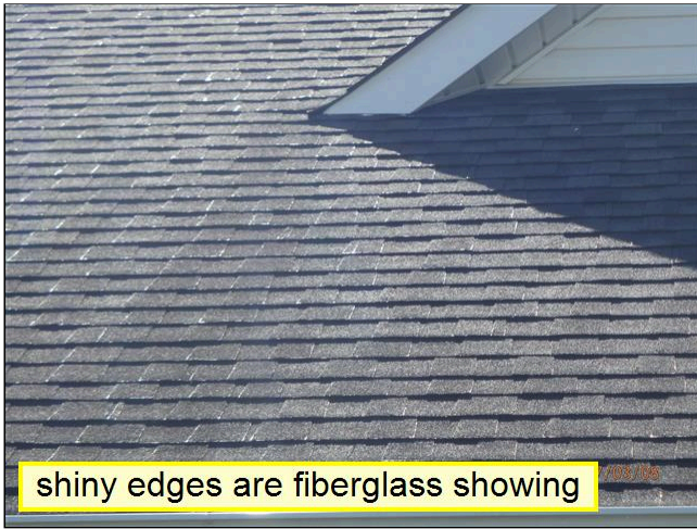
1.0 ROOF COVERING (.1) Item 3(Picture)
