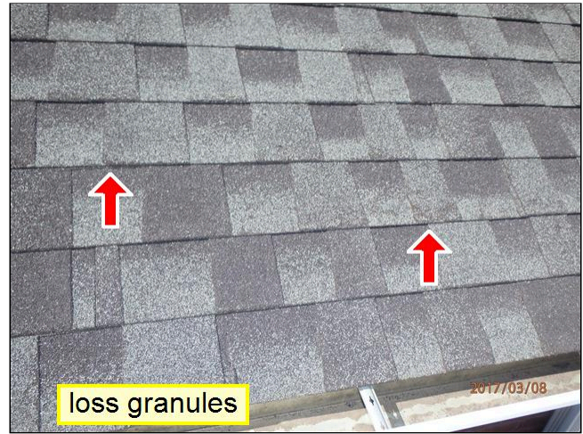
1.0 ROOF COVERING (.1) Item 4(Picture)
