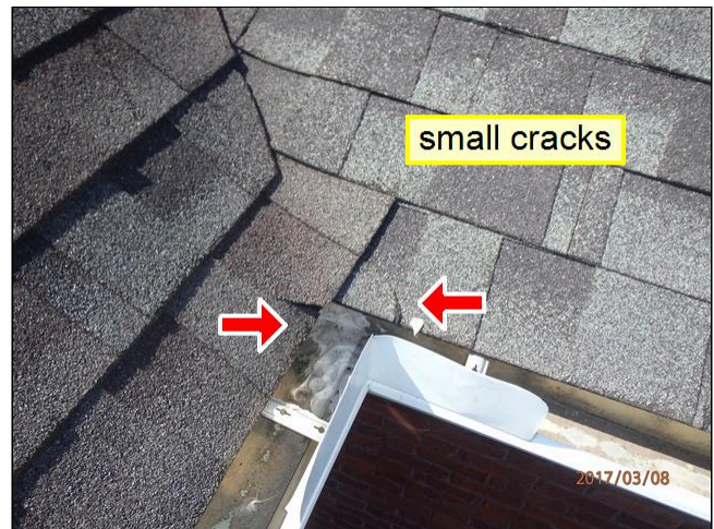
1.0 ROOF COVERING (.1) Item 2(Picture)
